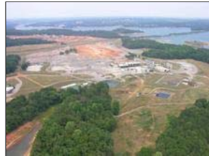
It's being called the biggest thing to hit Oconee County since the nuclear station and Keowee Key and it's going up on the site of what was the biggest thing in Oconee County. Gone is the Clemson Plant or Clemson Complex of the former J.P. Stevens Company, later known as WestPoint Stevens. The giant complex, like most of America's textile manufacturing, fell victim to the declining textile market in the United States and cheaper labor outside the country.
